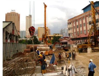
2012 - CBP, BP, Cavity Treatment In Limestone Substrata - Mercu Zikay, Kg Baru
