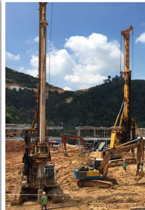
Apartment KTN At Lot 59191, Hulu Langat
